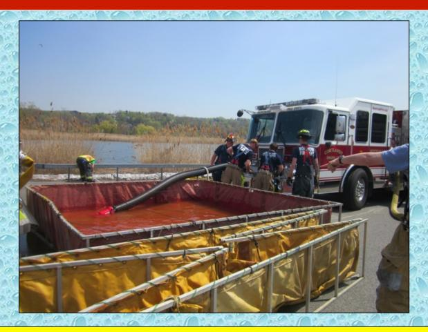
With the first tank down, a second dump tank is dropped off in anticipation of expanding the operation.
