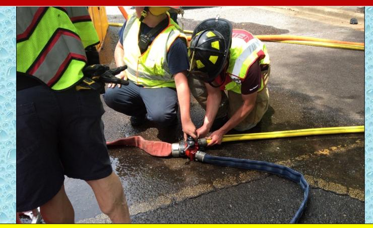
Control of the jet siphon water transfer devices was moved remote from the dump site pump operator in order to have better control over the water transfer process.
