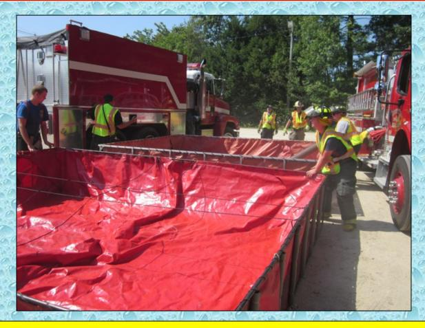
A second dump tank is put into place around the 3:46-minute mark in preparation for expanding the operation.
