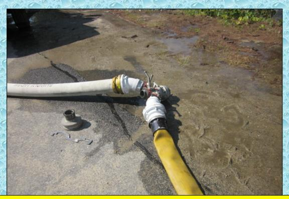
While this loading station arrangement was not pretty, is was quite functional in that the tankers were loaded quickly using LDH - while at the same time, the hose could be drained in order to disconnect from the tanker's direct fill in as short a time as possible.
