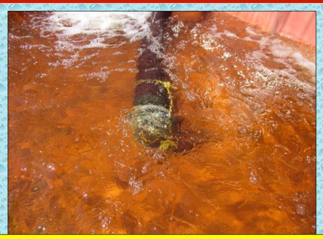
The low-level strainer was replaced with a 6-inch, basket-style strainer and the flow capability was instantly increased to 1,100 gpm!
