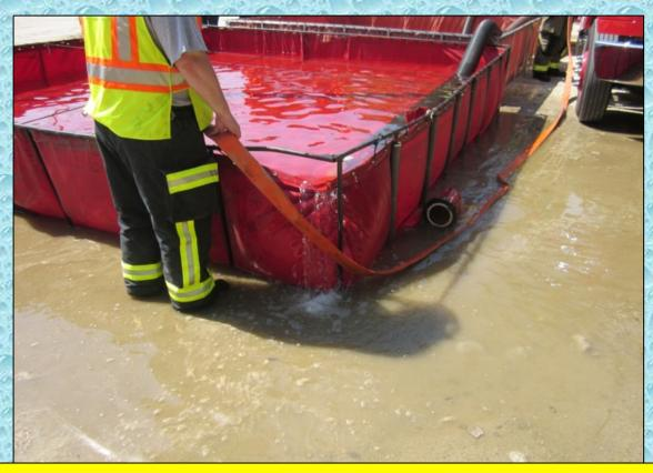
A slight problem occurred when the attachment rope broke on the corner of the second dump tank. Fortunately, the crew was able to repair the corner so that minimal water was lost.
