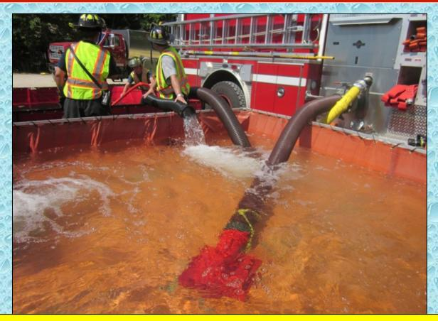
As usual, water transfer operations were critical to the success of the operation. Jet siphons were used to make the transfer of water from the outer tanks to the primary drafting tank.
