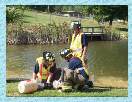
Only one floating strainer – but two suction lines? No problem – make your own floating strainer. Engine 203's crew uses an empty foam bucket as a float for a barrel strainer – thus – a floating strainer. It worked just fine!
