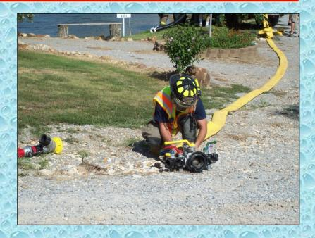
Brierfield Engine 203 was the first pumper to arrive at the pond fill site and the crew made quick work of getting a fill station set-up. A 5-inch supply line was layed from the loading area back to the drafting area and the line was trimmed out with an LDH manifold.
