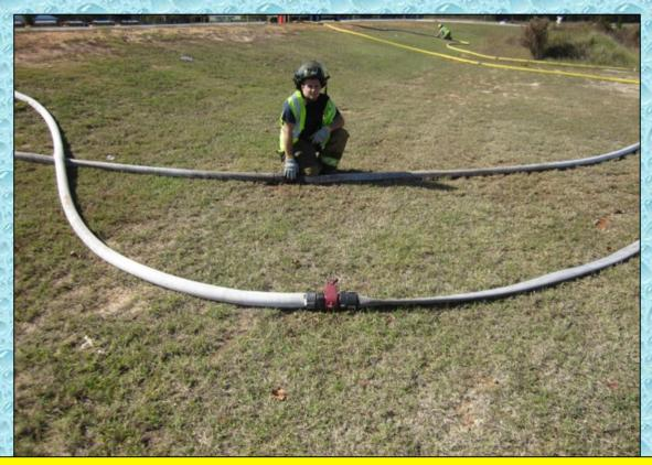
In-line gate valves were used as fill control valves. The use of a valve on a tanker fill line is important because it reduces the need for a pump operator to open and close pump control valves.
