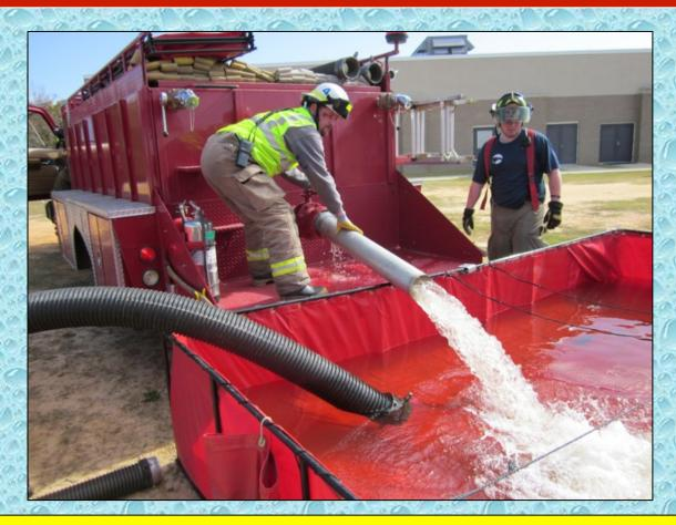
While still just using one dump tank, the next tanker arrives and dumps its 1,500 gallons of water.
