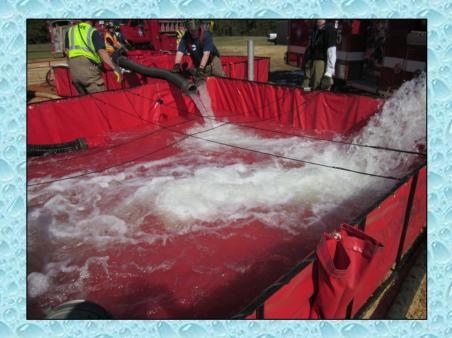
The water flow was NEVER lost at the attack pumper during the drill. But...at the dump site, it was very close to running out of water near the end of the drill. Fortunately, a tanker arrived just in time to sustain the operation. The 750 gpm flow rate was the maximum that this arrangement could support.
