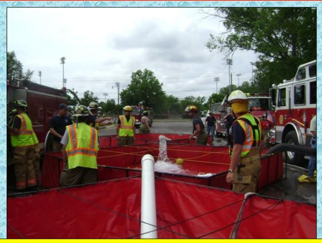
With three dump tanks now in position, Brierfield folks use two of their homemade 6-inch PVC jet siphons to begin transferring water.
