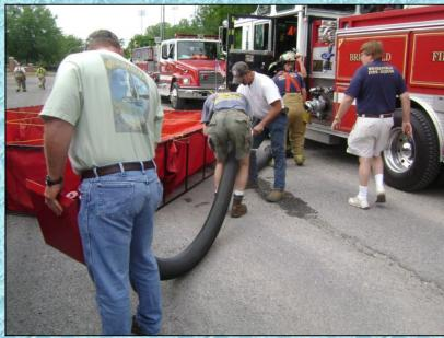
Meanwhile, crews hustle to build out the dump site. Suction hose is connected to Engine 202 (1,500 gpm) which will serve as the dump site pumper.
