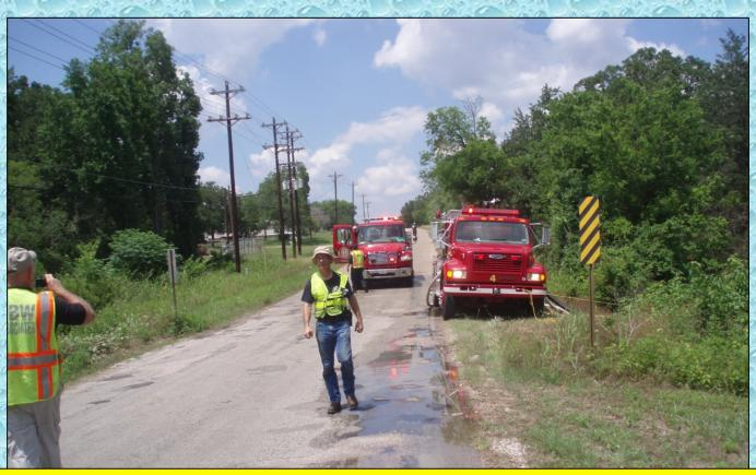
Smithville Engine 4 (1,250 gpm) established a draft where water passed under the road through a culvert. The lift was less than 10-feet and the water was clean and plentiful.
