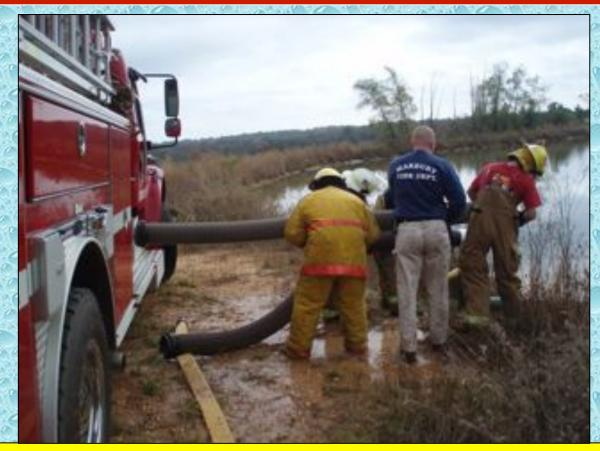
Another issue that arose was a leak at one of the suction hose couplings requiring the hose to be changed out in order to obtain a draft.
