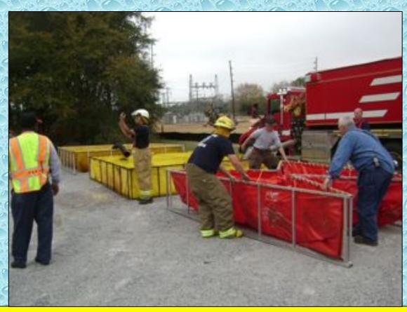
A third, 3,000-gallon dump tank arrived and was set up in preparation for expanding the flow.
