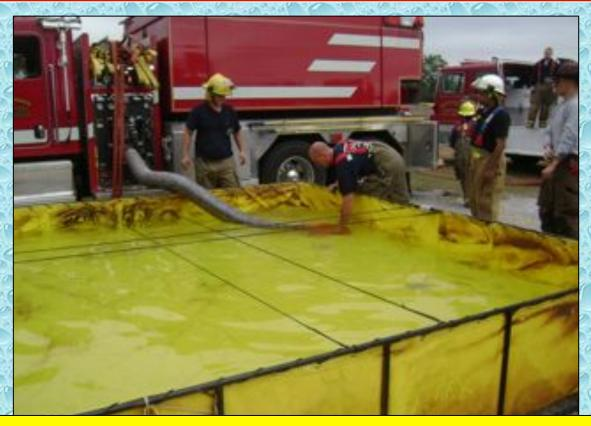
With the dump tank now in operation, the flow was restored to the attack engine and work was started on getting a second tank set up. By keeping the 3,000-gallon tank on Engine 901 full, this served as another dump tank – just on wheels.
