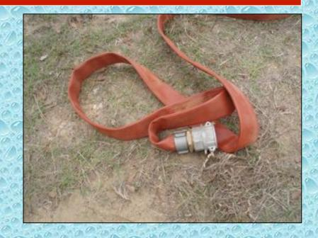
Two, 3-inch lines were stretched back out to the road to serve as tanker fill lines. The lines were trimmed out with camlock fittings in order to speed up the connecting and disconnecting operations.
