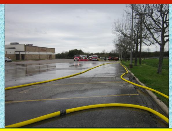
One of the challenges was overcoming the friction loss in the supply hose. In order to hit the 800 gpm mark, a second, 3-inch supply line was hand-laid back to the supply pumper.
