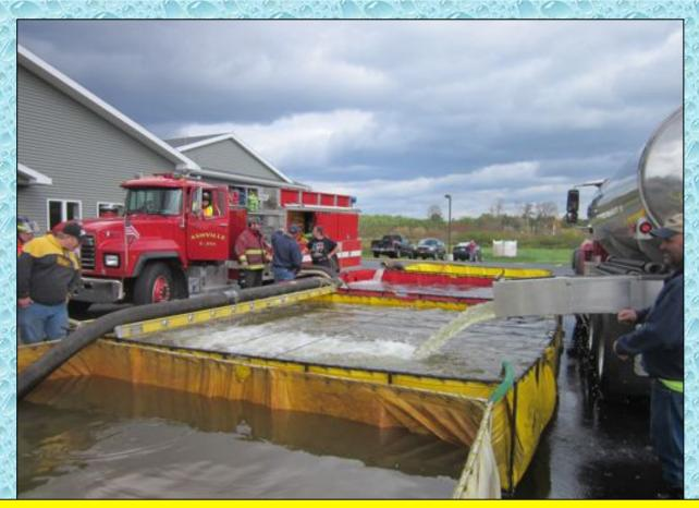
At the 30:00 minute mark with all four dump tanks full, the flow was increased to 750 gpm.
