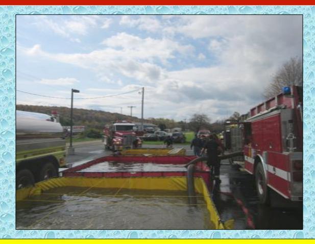
Three dump tanks in operation. The flow was moved to 500 gpm at the 15:00 minute mark.
