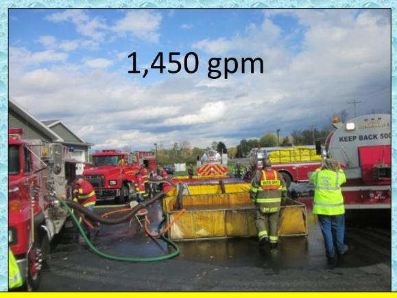
Flow was moved to 1,000 gpm at the 81:00 minute mark, to 1,250 gpm at the 108:00 minute mark, and once again to 1,450 gpm at the 113:00 minute mark – all without interruption!
