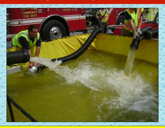
With a 1,000 gpm flow, water transfer operations were critical to the success.
