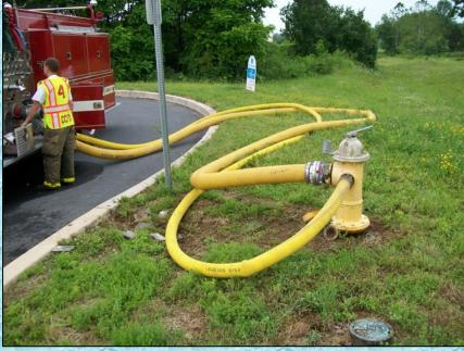
Cashtown's Engine 43 (1000 gpm) established a second fill site at a hydrant located on Expedition Trail. The crew did a good job of maximizing their water intake by using multiple outlets on the hydrant.
