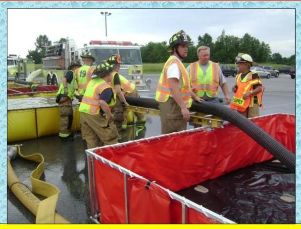
At the 50:00-minute mark, a 4<sup>th</sup> dump tank was added to the operation to help support the needed flow.
