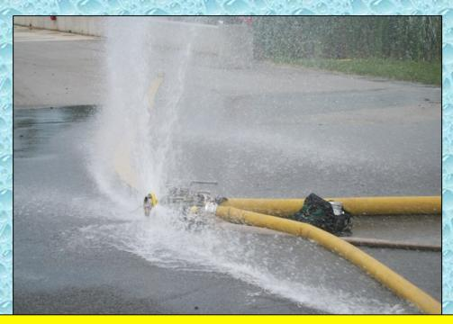
A problem occurred at one of the LDH manifolds being used at the fill site. The crew had set it up in reverse to serve as a large drain for bleeding off pressure when disconnecting from a tanker. However, they also set-up fill lines off of the 2-1/2" fittings — which defeated the purpose. To fix that, they placed a 5-inch cap on one of the 5-inch inlets. The bottom line is that the photo above shows what happened. The crew did remedy the situation however.
