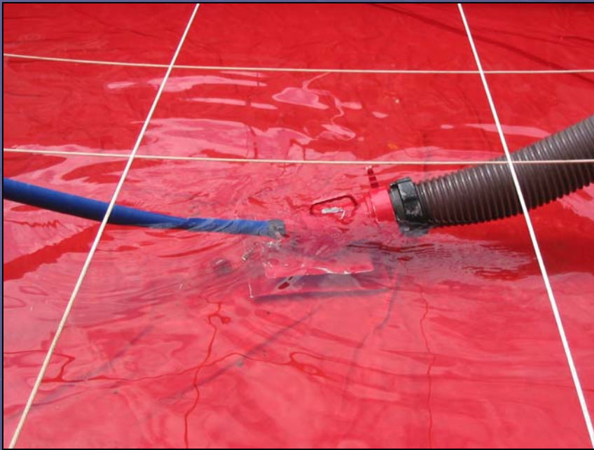
A Kocheck low-flow strainer with a built-in jet siphon.
