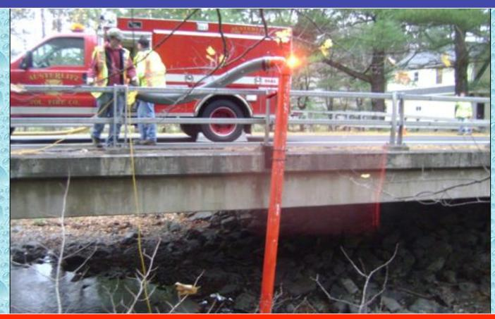
One of the concerns with this type of installation is the height of the suction head compared to the suction inlet on the pumper. At this installation, flow was not impacted even though the suction head was high.
