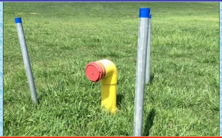
A 6-inch NST male suction head with an aluminum cap. When suction heads are exposed to mowers and vehicles, then protective bollards are recommended.
