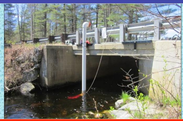
Like the others, once deployed, the standpipe system rests on the streambed and the standpipe carries the load.
