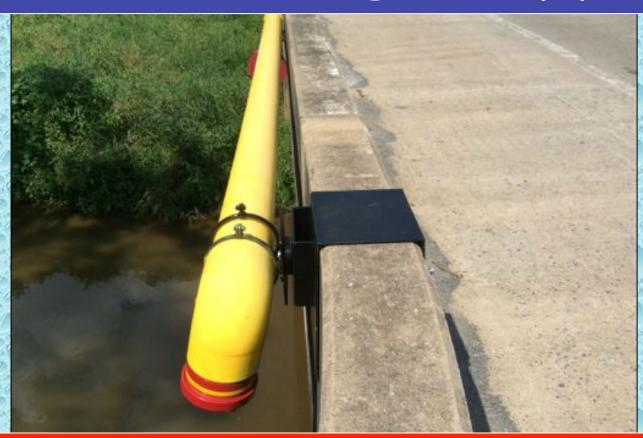
The standpipe is constructed of 6-inch PVC pipe and is outfitted with a tear drop style strainer and a 6-inch NST male suction head. A simple, rope retrieval/lowering system is used to maneuver the standpipe.
