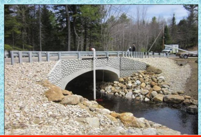
The lift at this location was high, but not insurmountable. And...it was the only reliable water source in the area. Once deployed, the suction head was in position for FD access.
