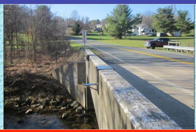
The saddle mount is the preferred mounting system for this style of bridge. The mounting system allows for a secure anchor while also adding flexibility if the location has to change in the future due to stream flow changes.
