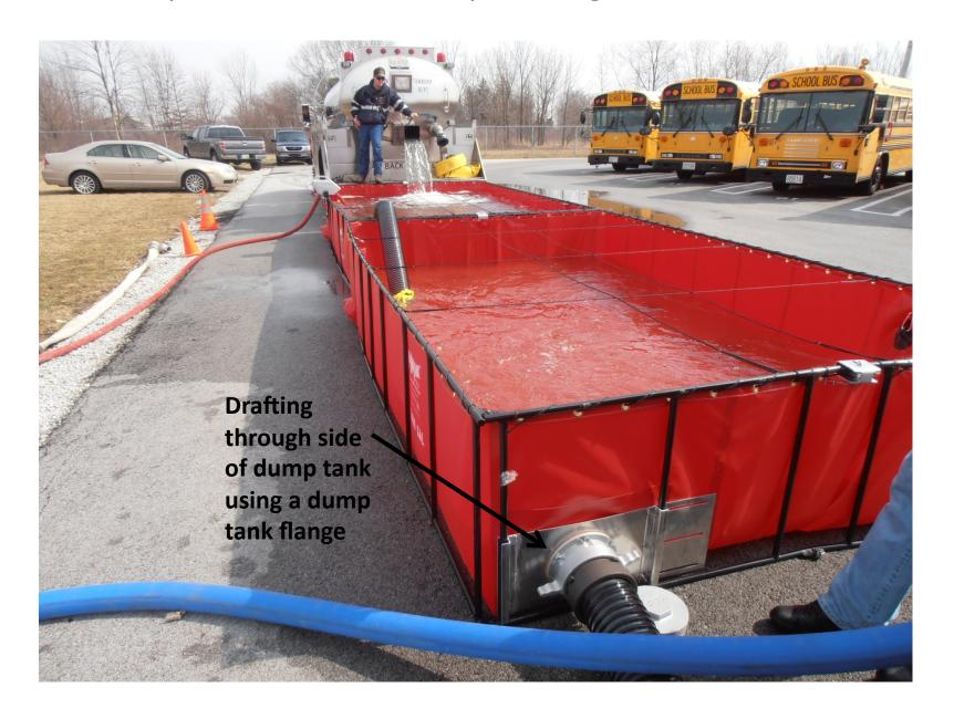
The low level strainers were attached to the dump tank flange inside the dump tank.
