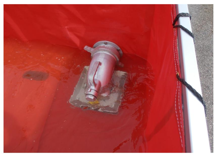
A 90 degree suction elbow guides the 6 inch suction hose down along the running board of the pumper.
