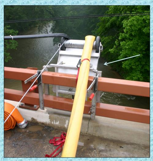
Once deployed into the water, the pump was powered up and the 4-inch hose charged. The hose had to be tied off to prevent additional hose from being pulled over the bridge railing.
