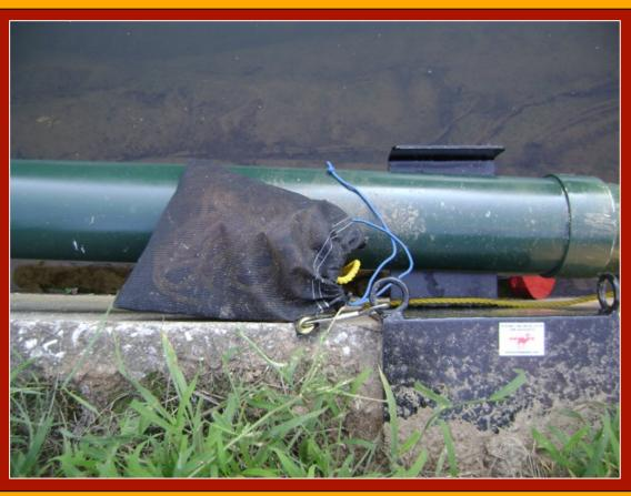
A polypropylene rope is attached to the strainer end (the eye bolt installed earlier) and stored in a mesh bag until needed.
