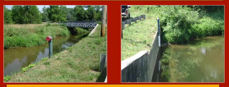
Storm debris from a flash flood destroyed the existing, "fixed-mount" dry fire hydrant that had been in place for many years. The debris tore off the lower part of the suction pipe – including the strainer. GBW Associates, LLC was contracted by the Water Resources Committee of the Baltimore County Volunteer Firemen's Association about replacing the damaged hydrant with a GBW swivel mount system.
