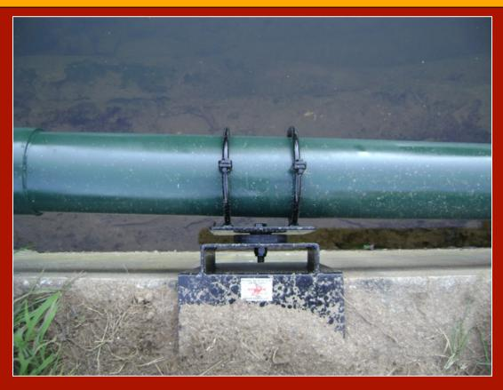
With the pipe now affixed to the swivel bracket, the system can be rotated and placed into the "stowed" position.
