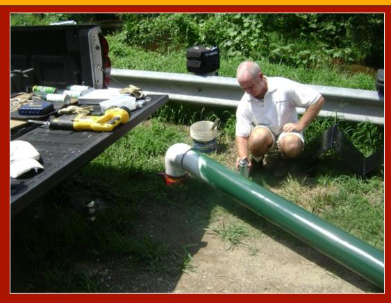
Painting is important in order to extend the life of PVC pipe exposed to the sun's ultraviolet rays.
