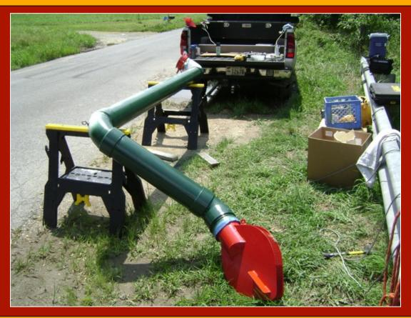
For this project, the exposed PVC pipe and fittings were spray painted green using a special spray paint designed for outdoor plastic materials.
