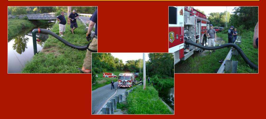
The final step of installation was a flow test. Jacksonville VFC Engine 473 (1,500 gpm) drafted from the new DFH and attained a flow of 1,012 gpm.
