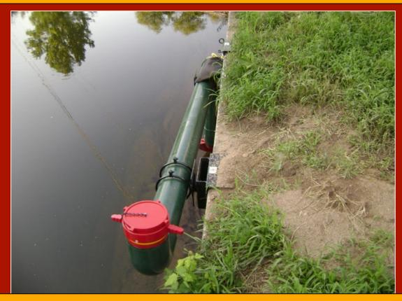
The final assembly. The pipe is stowed out of the water until such time that it is needed. When that time arrives, the pipe is swiveled into position and lowered into the water.
