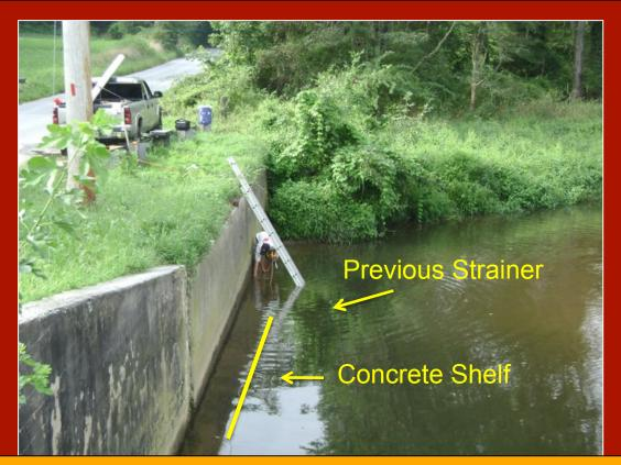
The concrete abutment posed a bit of a challenge because of a concrete "shelf" that extended out about 2-feet just under the water level. This shelf required a bit of an adjustment to the standard GBW design.
