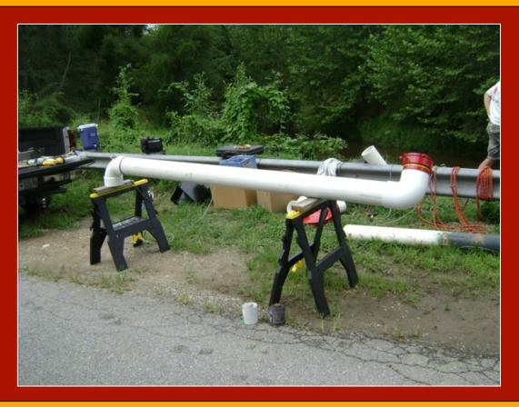
Now it was time for the final assembly of pipe – this meant more gluing followed by painting.
