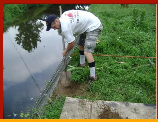
The next step – prepare the abutment to accept the swivel mount bracket. The device used a "non-destructive" mounting system – so no drilling or bolting was needed.
