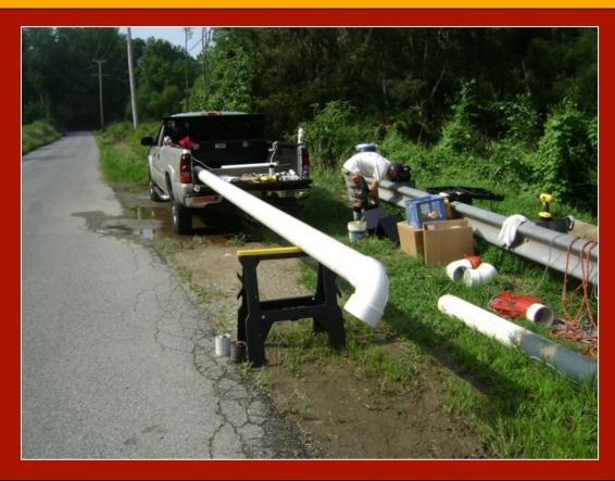
Meanwhile, pipe assembly is underway. This project used Schedule 40 PVC pressure pipe and fittings.
