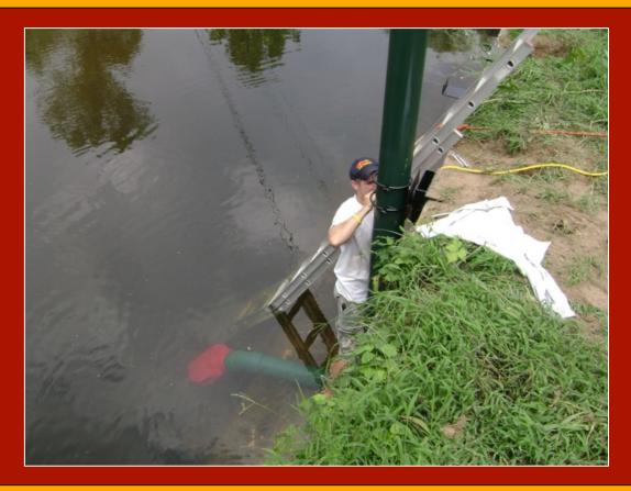
With the paint dry and the pipe ready for installation, the next step was to attach the pipe to the swivel bracket.
